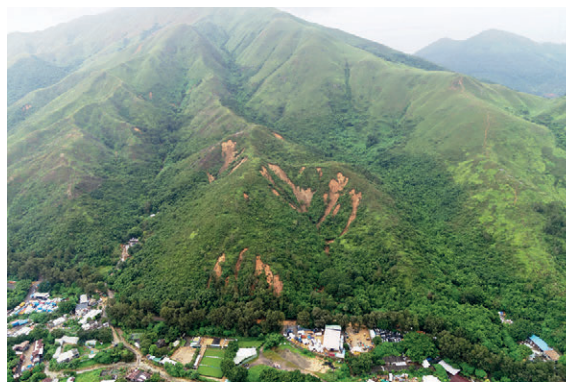
Rainstorms increase the landslide risk of natural terrain
