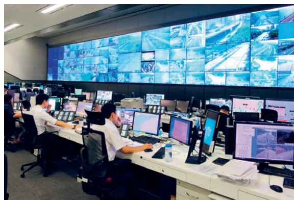
TD's Emergency Transport Coordination Centre monitors traffic conditions and handles various emergency situations
