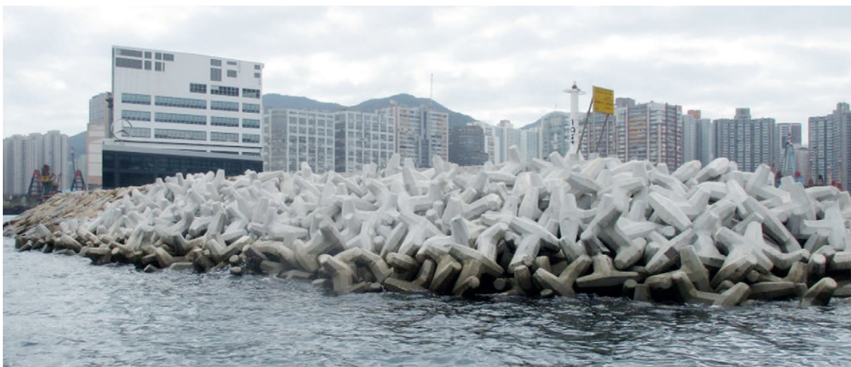
Chai Wan Breakwater
