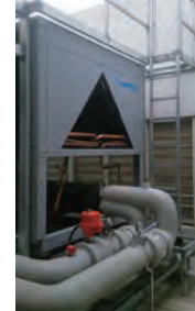
High efficiency air-cooled chiller
