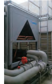
High efficiency air-cooled chiller
