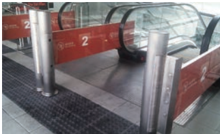
Service-on-demand escalators with passenger sensing post
