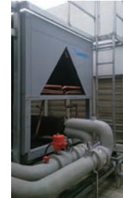
High efficiency air-cooled chiller
