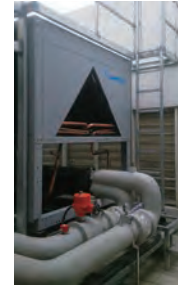
High efficiency air-cooled chiller
